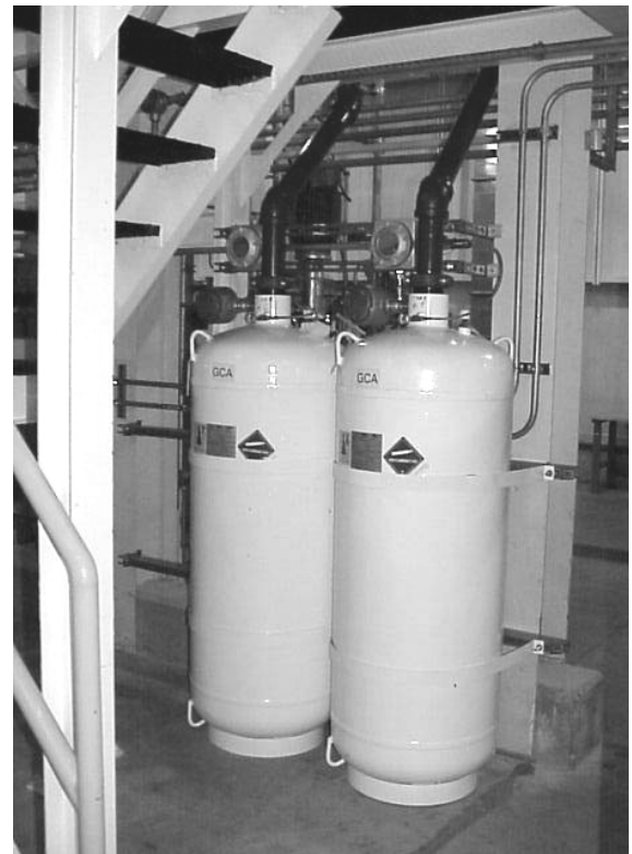
Fike HFC-227ea System Protecting a Flammable Liquid Storage Facility
